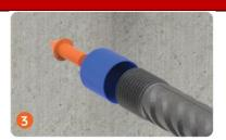
Remove the protection from the 2nd Phase bar.
